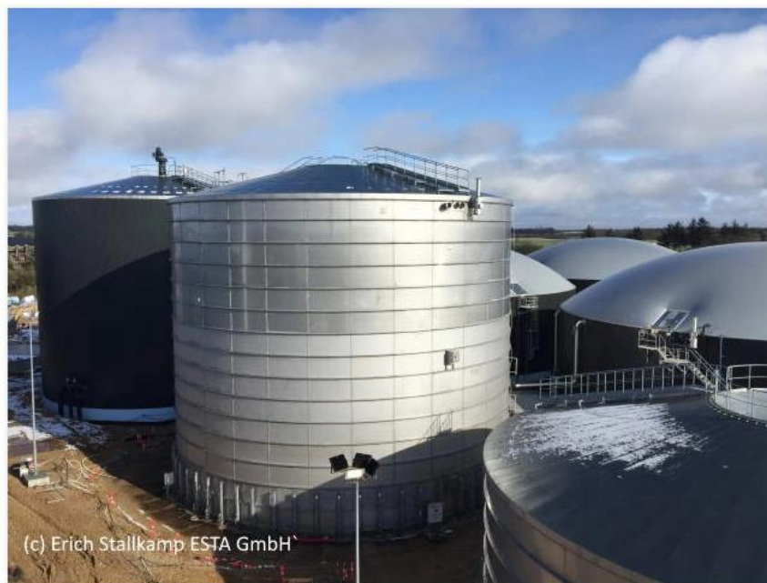
Stallkamp's tall digester CSTRs have a diameter of 15 m and a height of almost 20 m.
